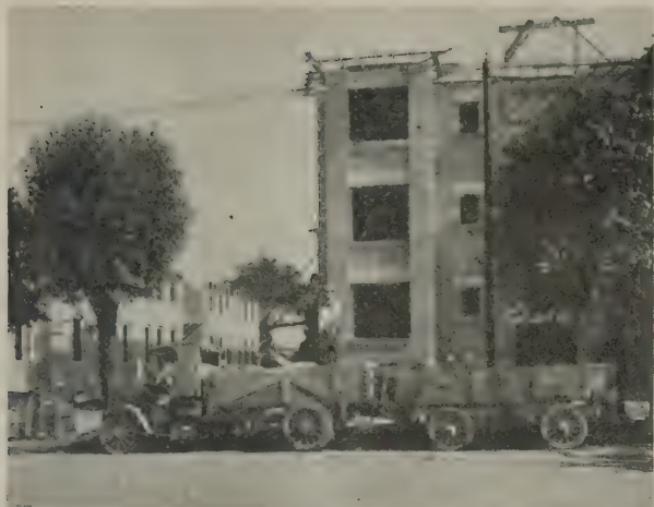
By the use of these trailers hauling cost of brick was reduced from $1.70 to 95c. per thousand.
